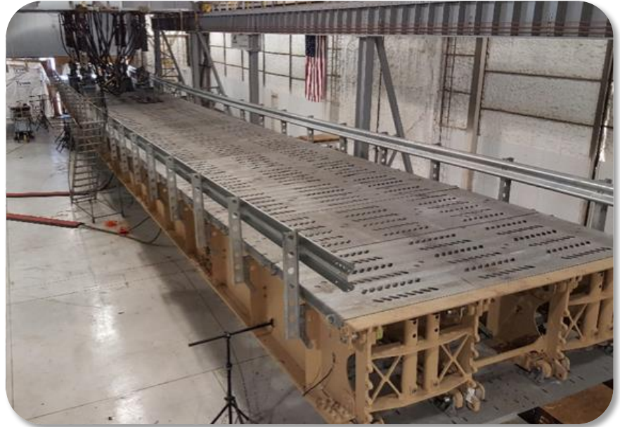
Long semi-permanent tactical bridge
